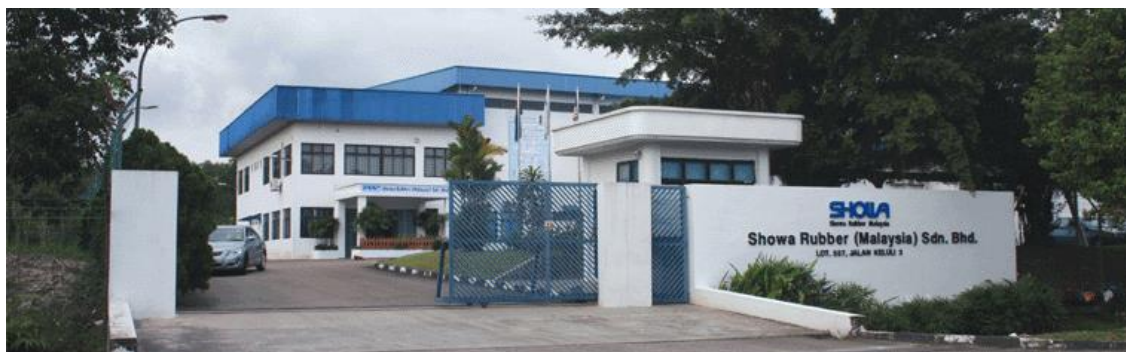
SRM Head Office and Factory located in Pasir Gudang, Johor, Malaysia
